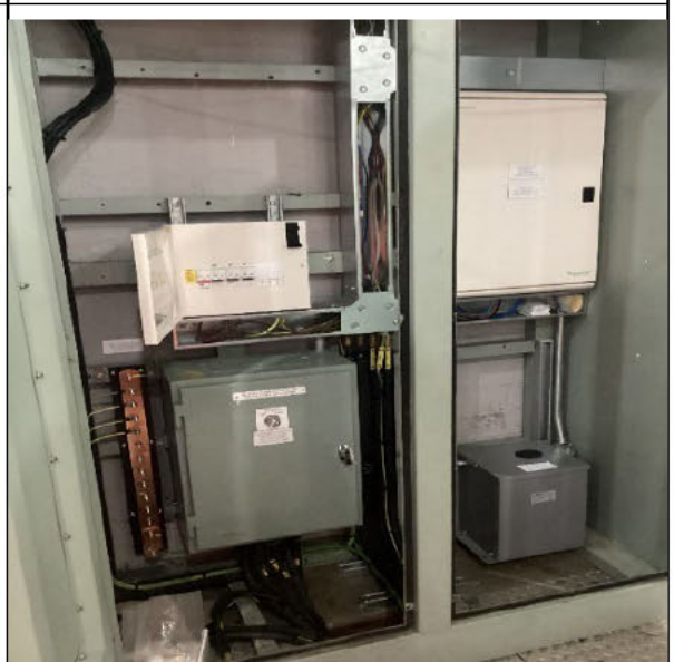
Figure 8: Post-replacement: DB LV and DB PL
