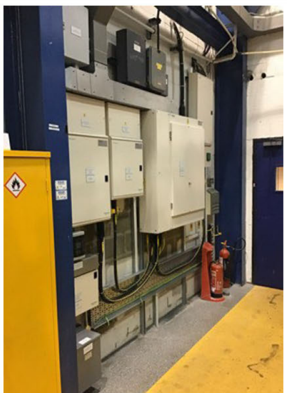
Figure 6: Post-replacement: DB H, DB E, DB G and Switchboard 3
