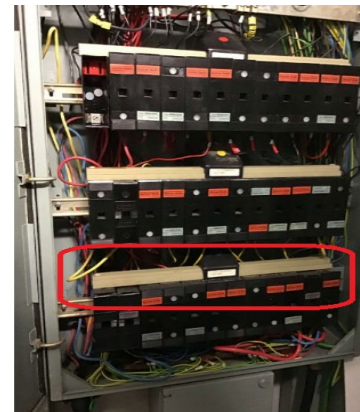
Figure 4: Services DB1 exposed terminations
