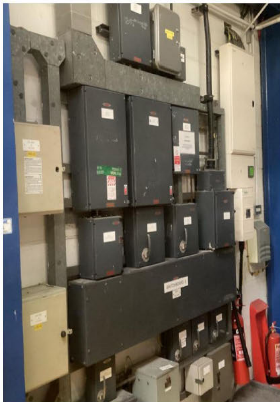
Figure 5: Pre-replacement: DB H, DB E, DB F, DB G and Switchboard 3
